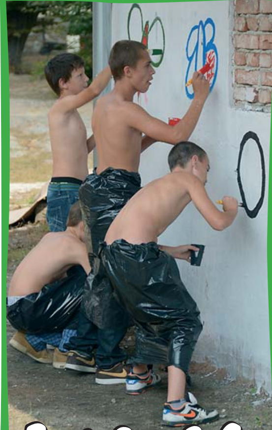
Volunteer Days 2011 – volunteers renovate the space of the NGO Garden in Banská Bystrica
