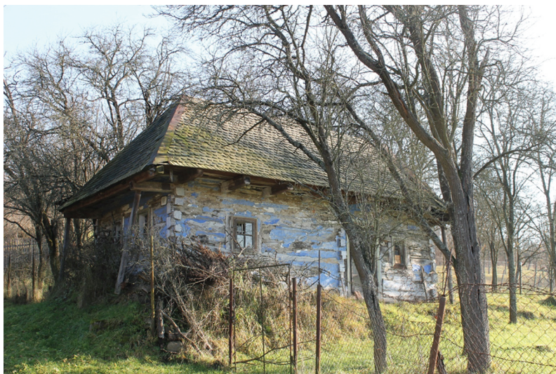
Figure 2. Abandoned traditional local models of dwellings in depopulated areas. Photo Ján Aláč.
